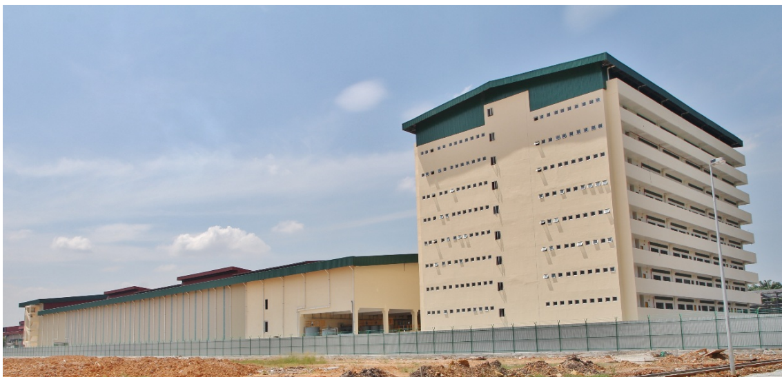
New Hostel for workers as part of CSR programme (picture taken on 23 August 2014)
