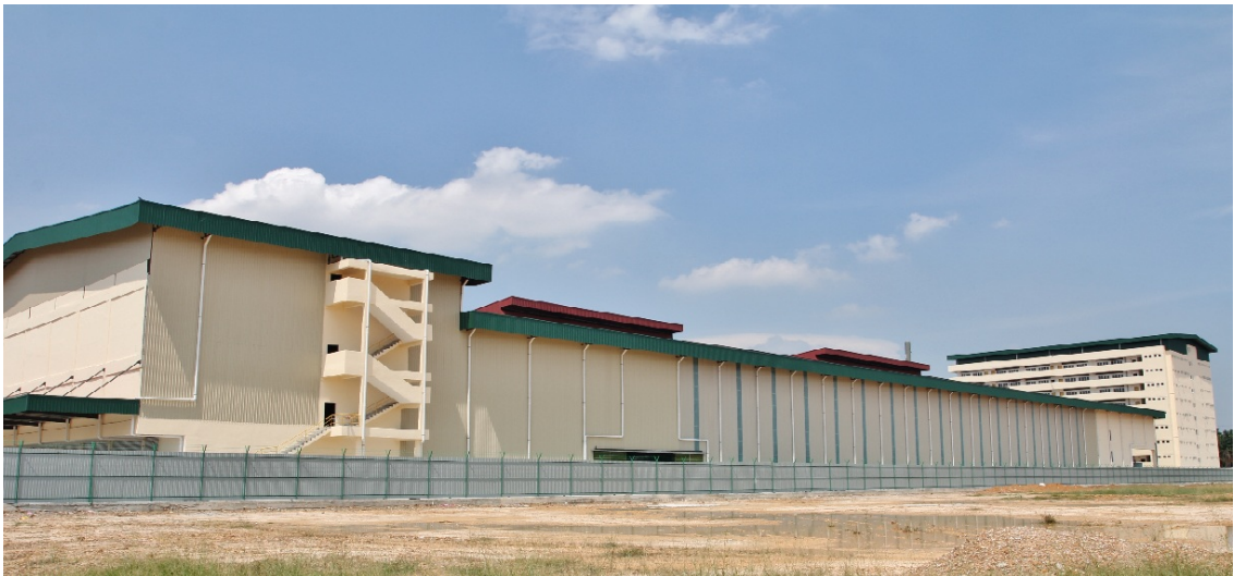
External View of newly-completed Factory No. 10 (picture taken on 23 August 2014)
